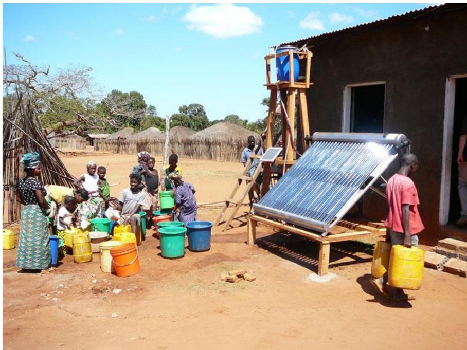
Fig. 1: The solar thermal water disinfection system installed at a testing site in rural Mocambique.
